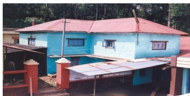
Fig. 5.36: Conventional cardamom curing chamber
